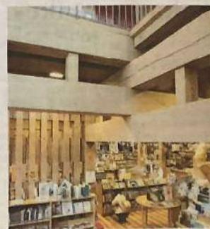
Two-tiered beams in the library
